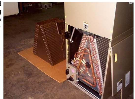
Air Handler with an un-coated coil and a coil coated with Bronz-Glow's Husky Coil Coat and Intersept to retard to the Dirty Socks Syndrome.
